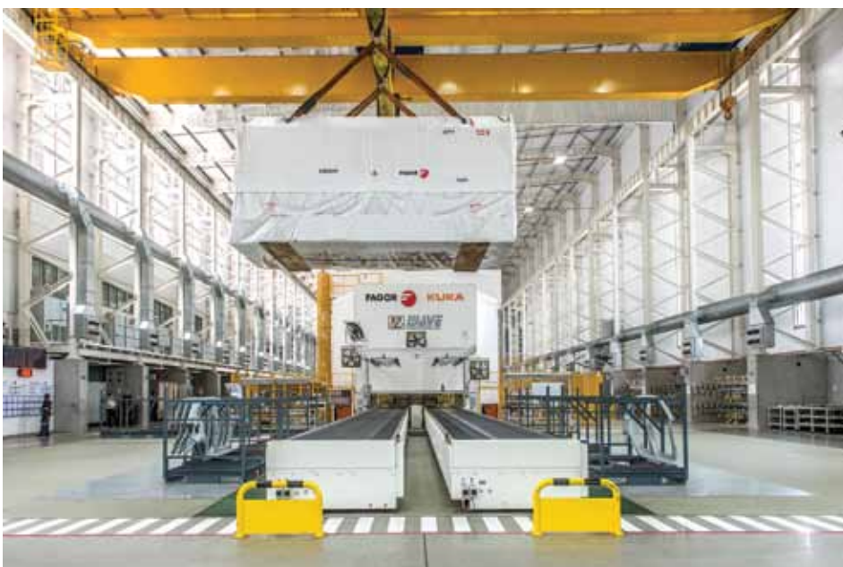
The press bed, weighing 120 tons was lifted 8 metres over the existing press line.
